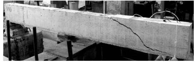
(a) Crack mapping [8]
